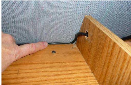
Figure 7. Camera cable goes through hole from wardrobe top into left tray.
